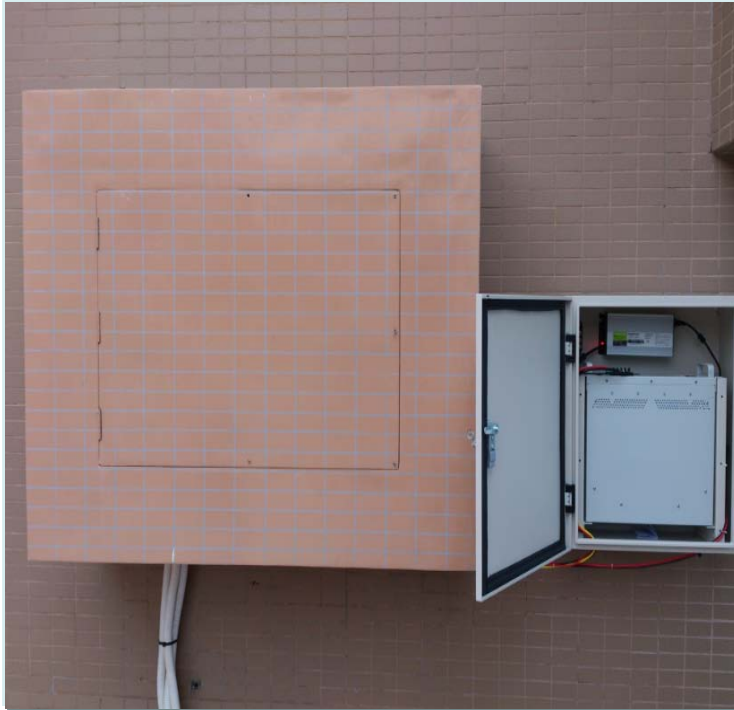
48V-50Ah Blocks—wall-mounted energy storage program of Unicom in Yangjiang City, Guangzhou
