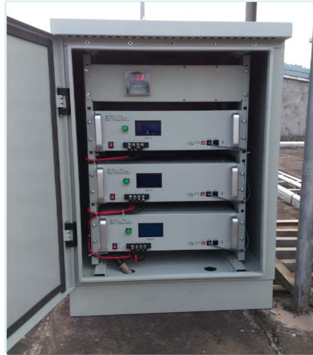
48V-150Ah Block—outside energy storage program of Telcom in Meizhou City, Guangzhou
