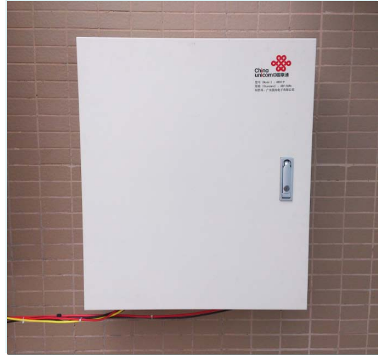
48V-50Ah Blocks—wall-mounted energy storage program of Unicom in Yangjiang City, Guangzhou
