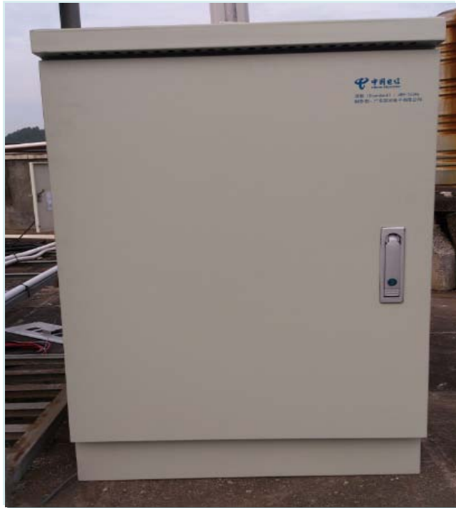
48V-150Ah Block—outside energy storage program of Telcom in Meizhou City, Guangzhou
